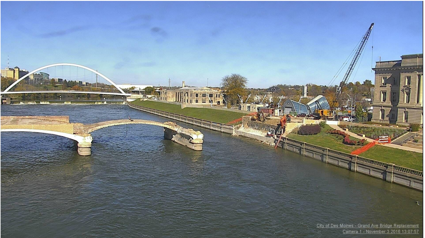
View Looking North-Northeast
