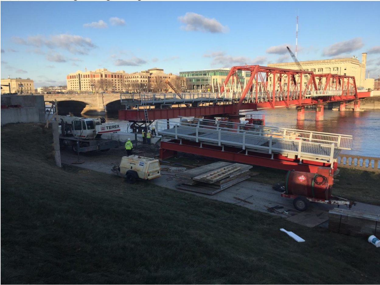
12/8/2016 Red Bridge Raising Starting This Month
