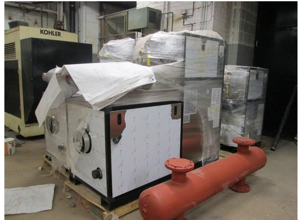
Three new boilers ready for installation.
