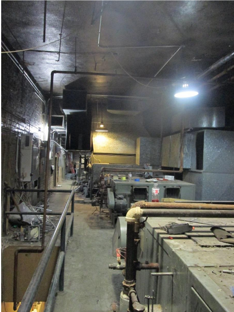
OLD MECHANICAL EQUIPMENT IN ATTIC
