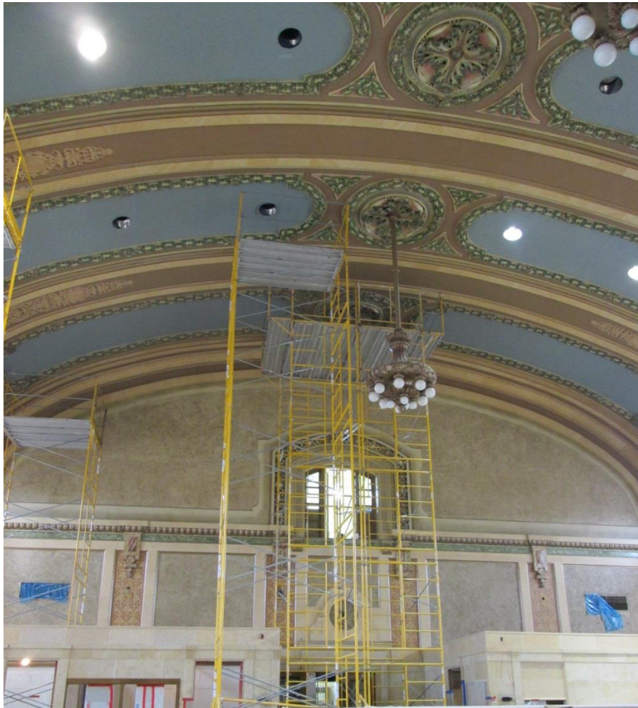
SCAFFOLD FOR SPRINKLER HEAD INSTALLATION IN THE GREAT HALL
